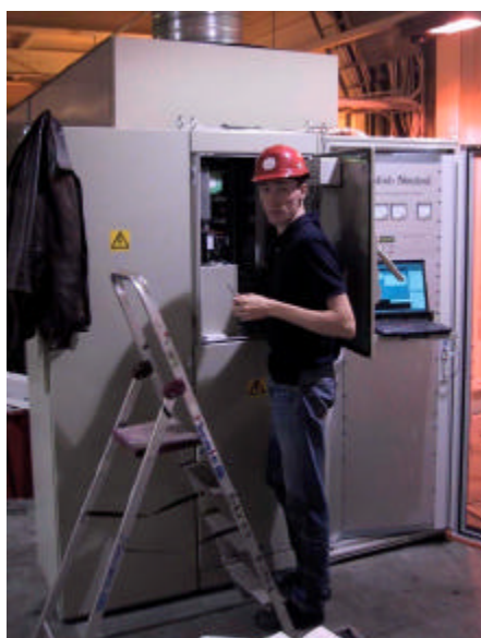
Figure 6: RCC Ground Fault Neutralizer, compact unit with integrated grounding transformer and arc suppression coil for industry applications
