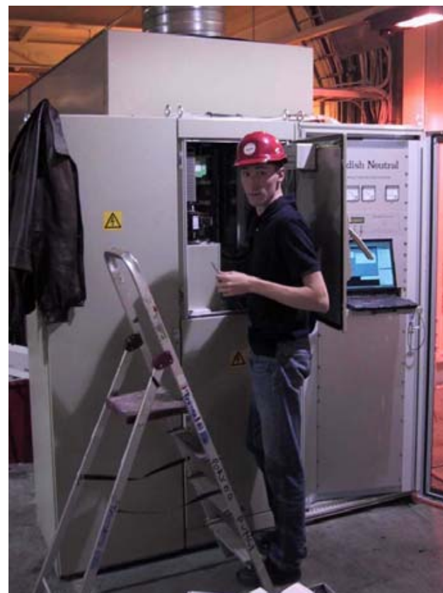
Figure 6: RCC Ground Fault Neutralizer, compact unit with integrated dry-type arc suppression coil for industry applications
